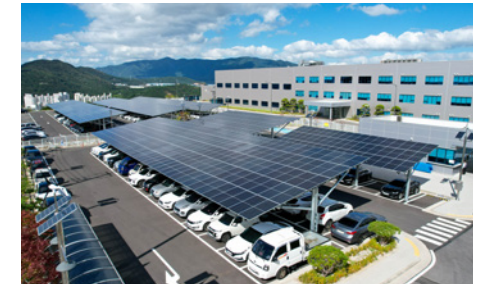
PV generators installed at the parking lot of the Ulsan Electrification Plant
